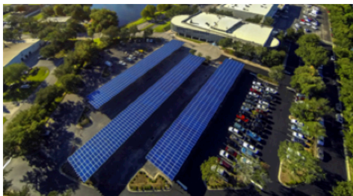
Figure 6 – Orlando Utilities Commission Carpark Community Solar Project (Source: Orlando Utilities Commission)
